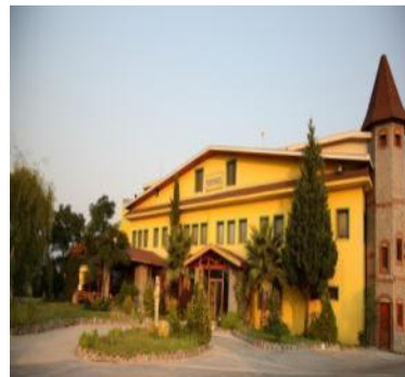
Inspection of the production unit
